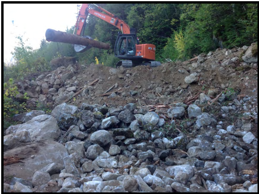
Town End Cribbing Removed
