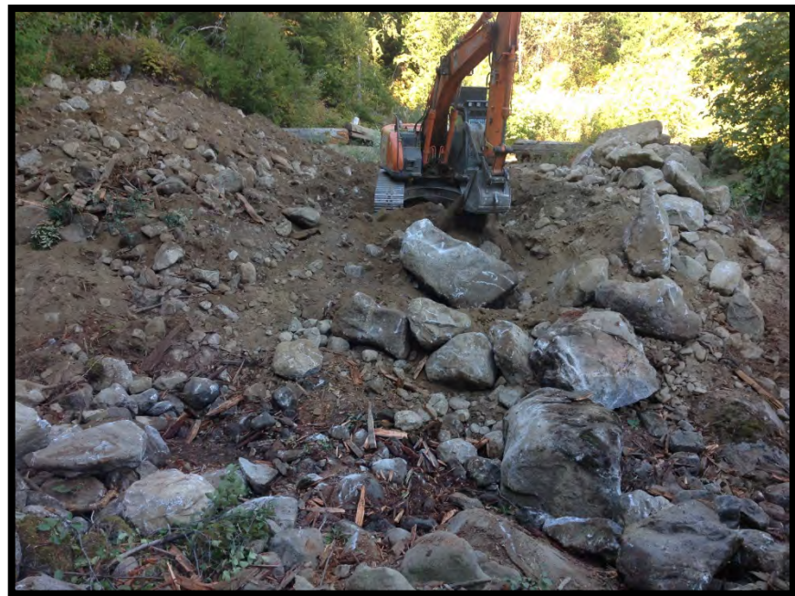
Large Boulders Encountered Excavating Approach
