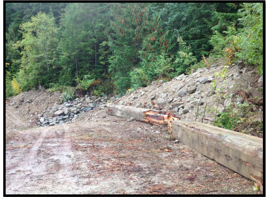
Surplus Excavated Materials – Sloped and Seeded
