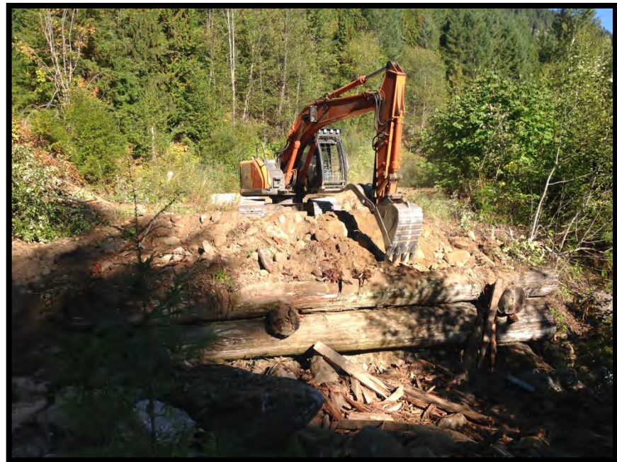
Stripping Road Fill from behind Cribbing
