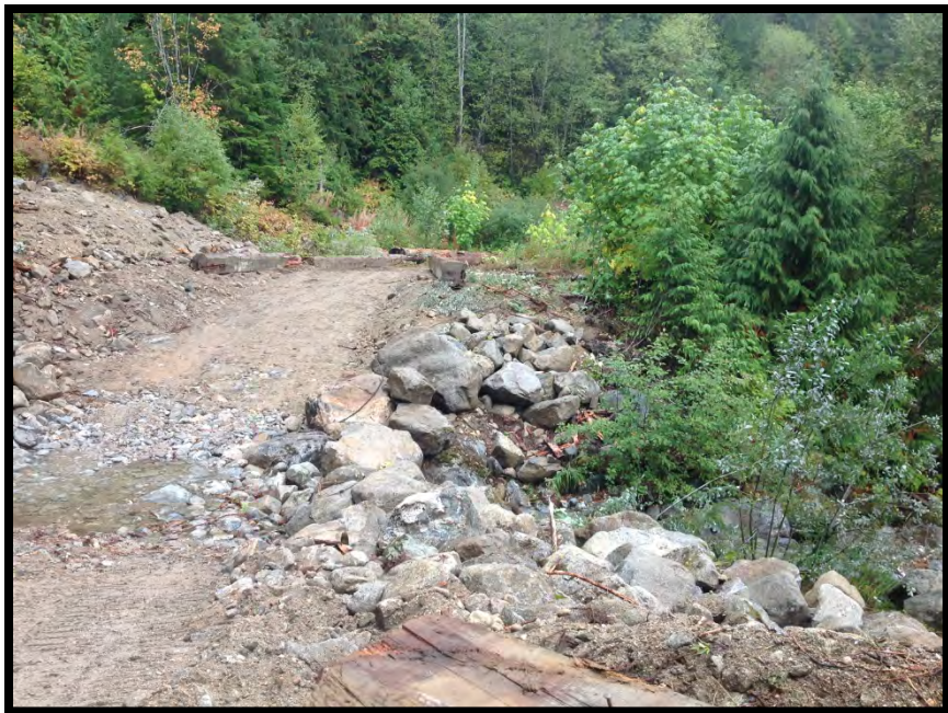
Large Boulders at Outlet
