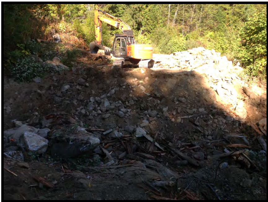
Woods End Cribbing Removed
