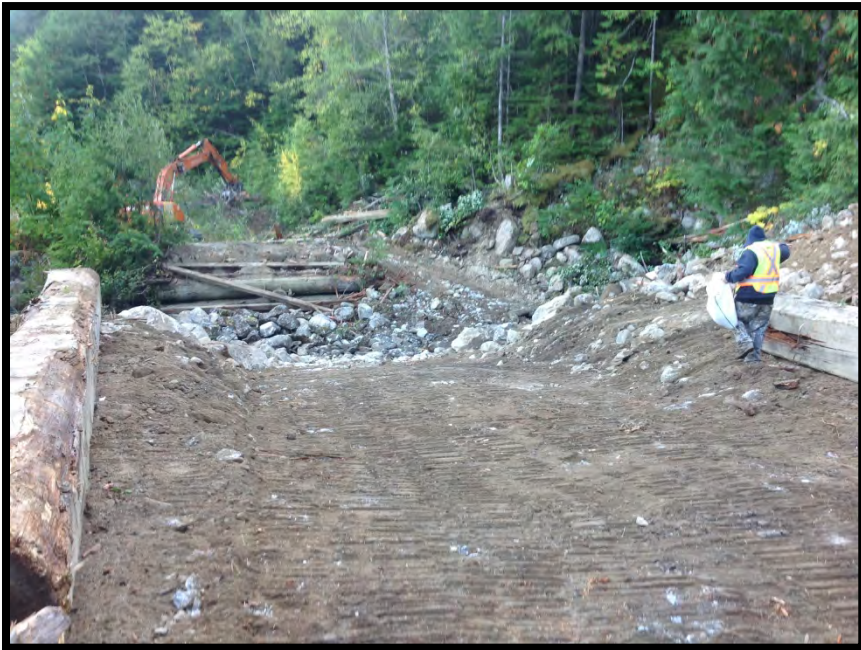
Grass Seeding in Progress
