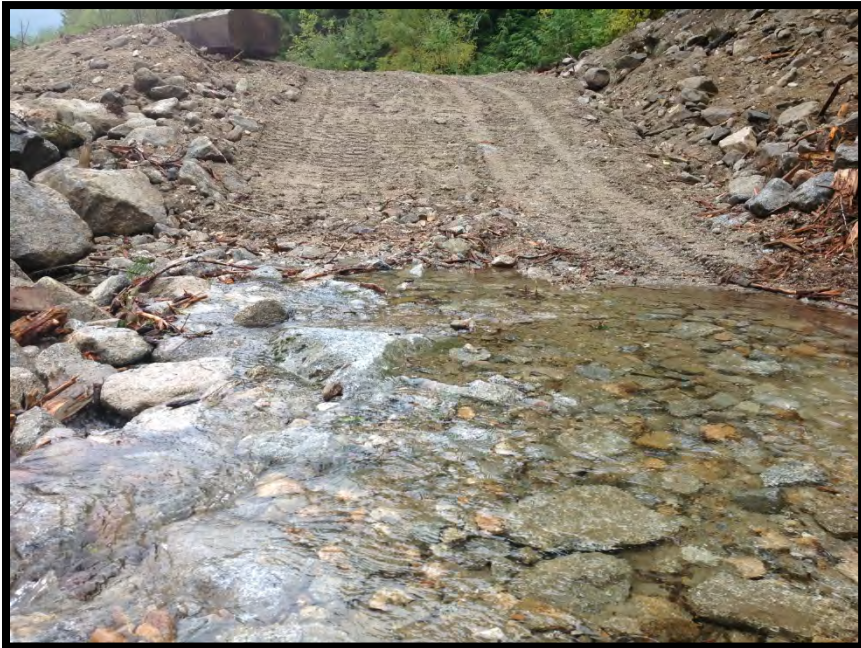
Large Boulders Embedded in Channel
