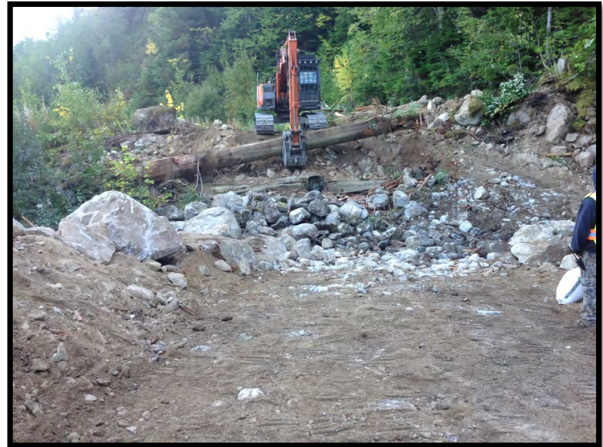
Town End Cribbing Coming Out
